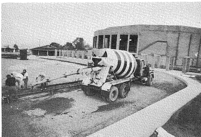
Finishing up the front curbs.
