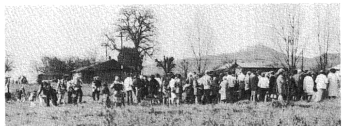
Ground-breaking - looking north.
