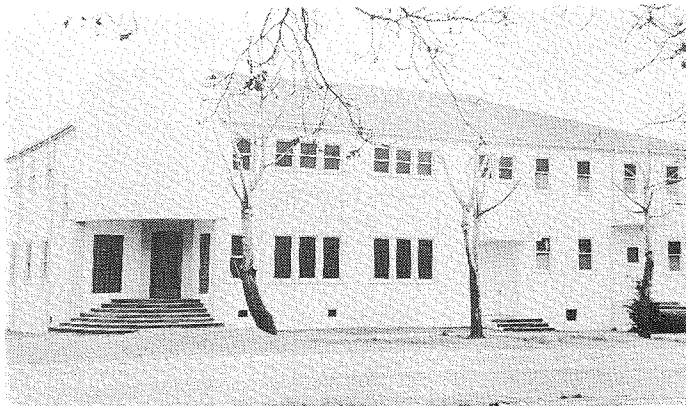
The finished building before sidewalks and pavement were poured.
