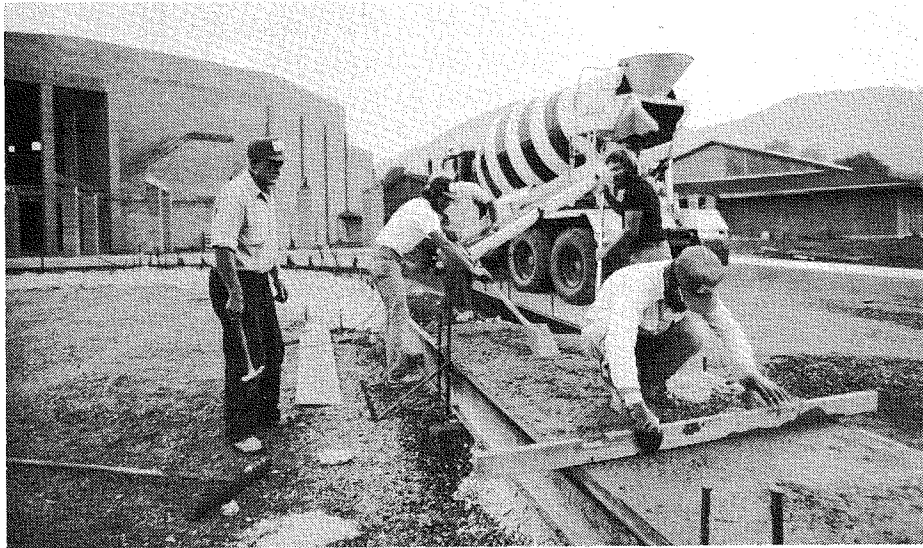
John Davison pours the front sidewalks for the new building.
