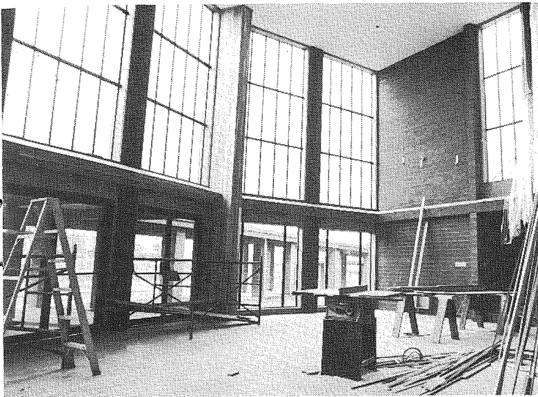
Narthex nears completion, January 2, 1978.
